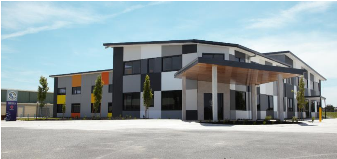
Stage 4F completed and ready for use in 2018 – 2400sq.m. of floor space – 15 classrooms and new Administration.
